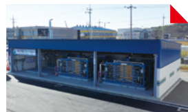
Completed the Hynet Hydrogen Shipping Center
